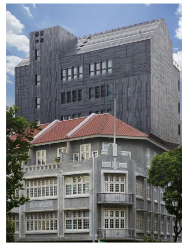
21 Carpenter comprises a four-storey conserved block of four shophouses dating back to 1936, with a contemporary six-storey rear block added. PHOTO: JOWIAN LIM
