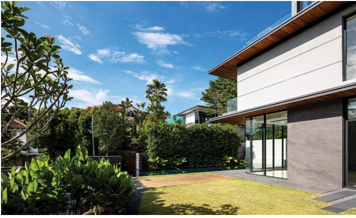
The lawn and swimming pool are on the first level, sitting above the basement carpark that can fit five cars
